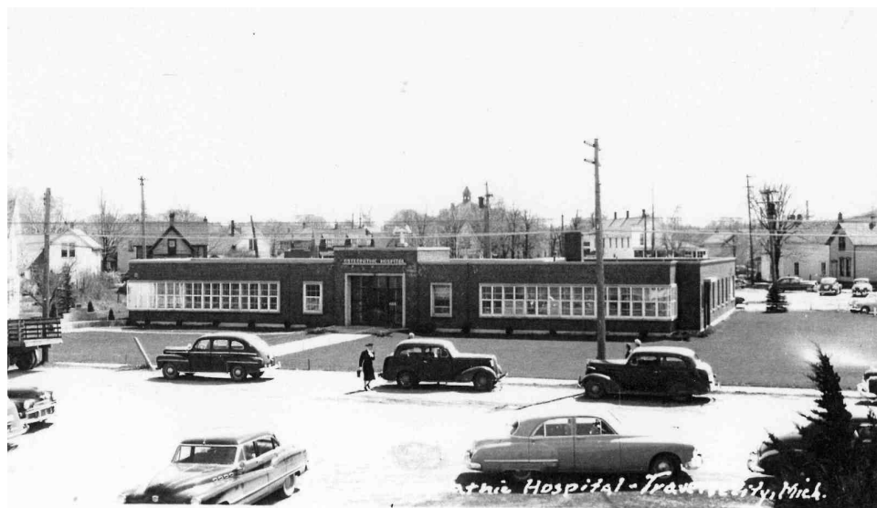
TCOH Bay Street Building
