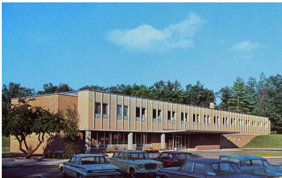
TCOH Munson Avenue Building
